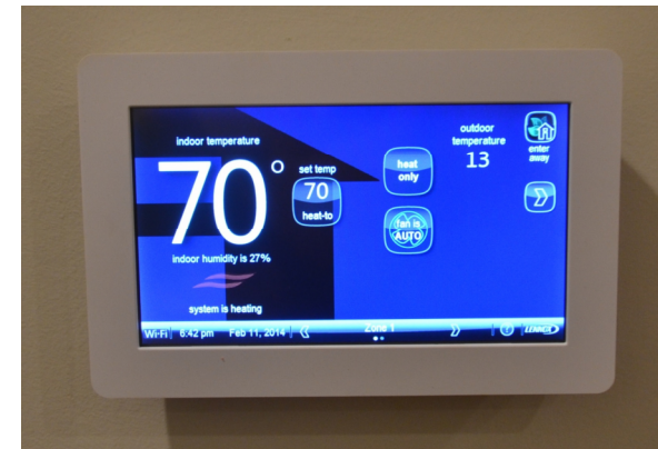
Building solution center
